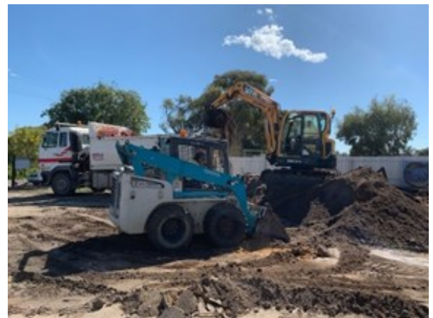
Back yard excavation
