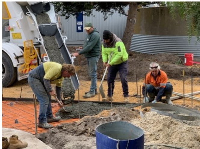
Concreting the kerbing
