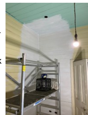
Primer on the wall ready for the Wi-Fi control box.
