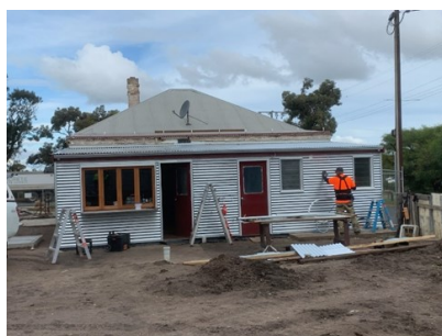
Dave fixing the last sheet in place.
