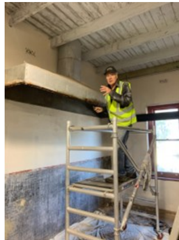
Phil treating the rust on the canopy
