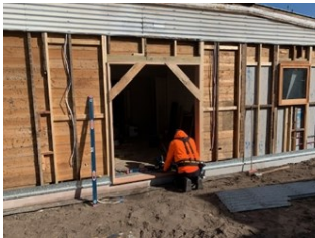
Dave installing the reception room door frame
