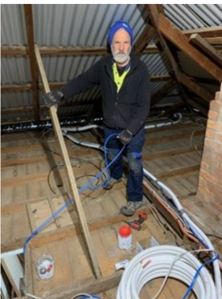
Grant in the ceiling
