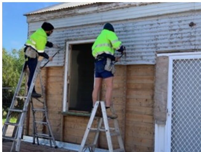
Removing the old cladding
