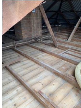
The cleared ceiling.
