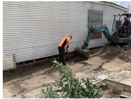
John Stratton clearing the footings with Dave's help.
