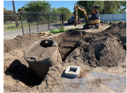
Removal of old septic tank
