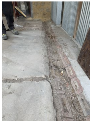
2 photo's showing our work on the trench
